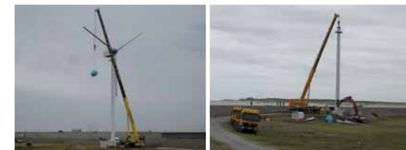
Demounting of the old ENERCON E-33 turbines at Roggeplaat Wind Farm.
