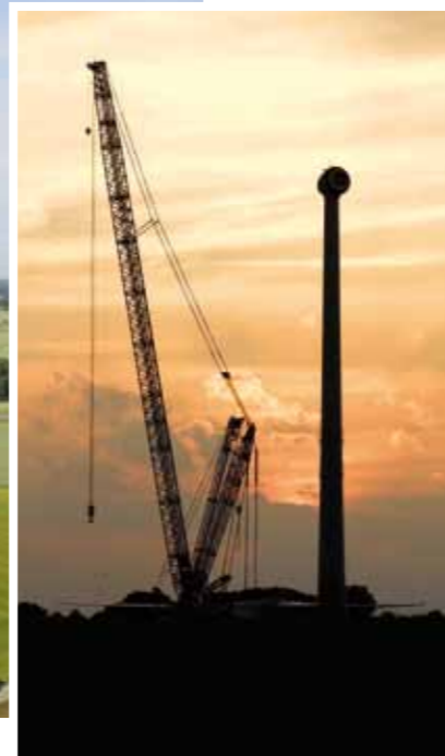
Mounting the E-101 machine house atop the 97-metre tower in Görmin.
