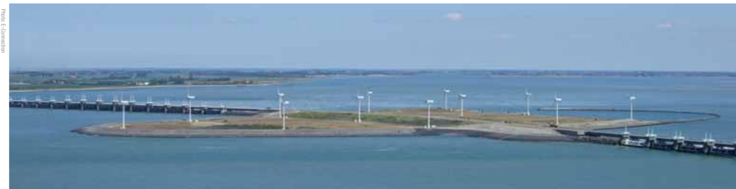
Roggeplaat at Oosterscheldekering is ENERCON's first wind farm abroad.
